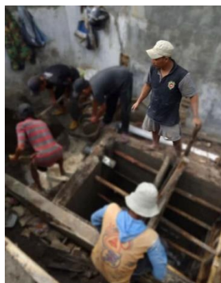
Figure 1.1 Construction of Toilets in Suci Village Source: (Researcher Documentation, 2023)
